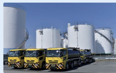
Storage tank & tank lorry
