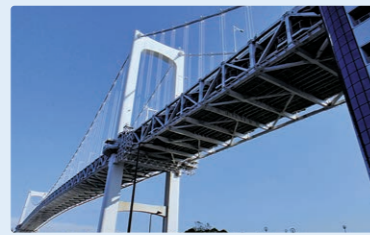
Rust proof paint
